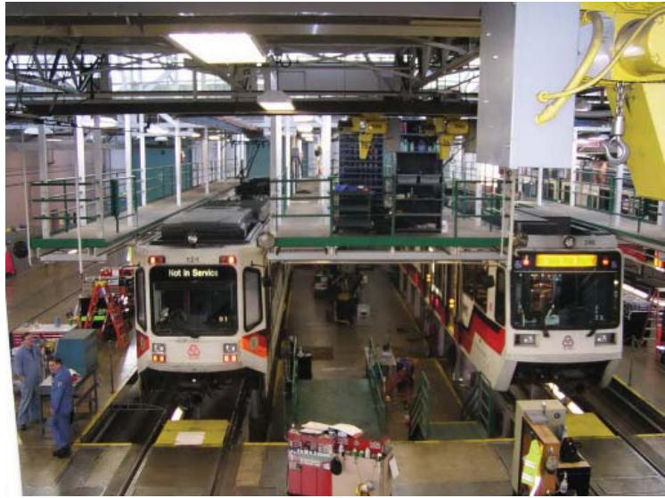
An example of a split-level facility specifically designed for servicing low-floor vehicles, Portland, Oregon. This type of design is based on the use of vehicles which have the majority of their propulsion and auxiliary components on the vehicle roof. By contrast, heritage streetcar vehicles have the majority of their equipment under the vehicle floor.
