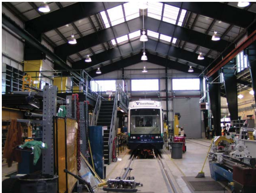
An example of a traditional facility outfitted with a platform to service roof components, Tacoma, Washington. If at some point in the future it were desired to utilize low-floor modern streetcars on the Red Car Line, the proposed facility could be retrofitted with similar roof-level platforms.
