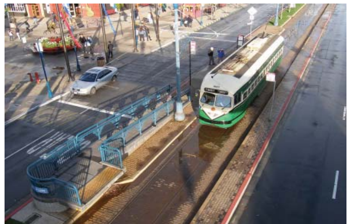
Streetcar stop with mini high-block and ramp, San Francisco, California. Streetcar is stopped at regular boarding area in this picture, and would pull up to ramp to board wheelchairs.
