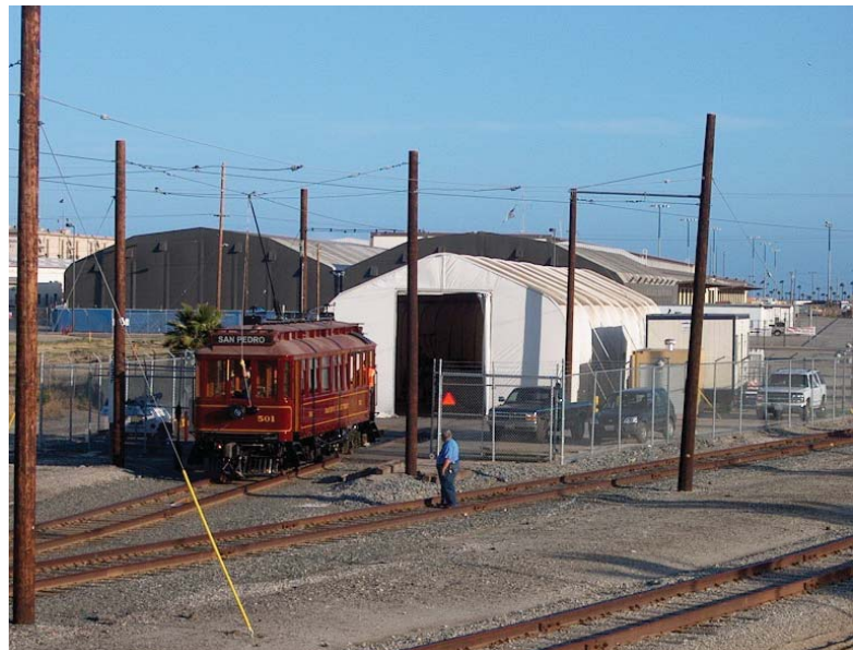
Existing Red Car Maintenance Facility. This temporary facility consists of a large tent and outdoor inspection pit, with office trailers and storage containers.
