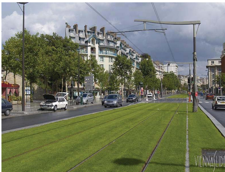
The appearance of the Red Car right-of-way can be enhanced significantly with "green" turf-track construction, commonly used in Europe.
